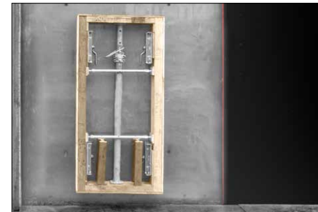
Box outs Magnets used to attach box outs and triangular filllets.
